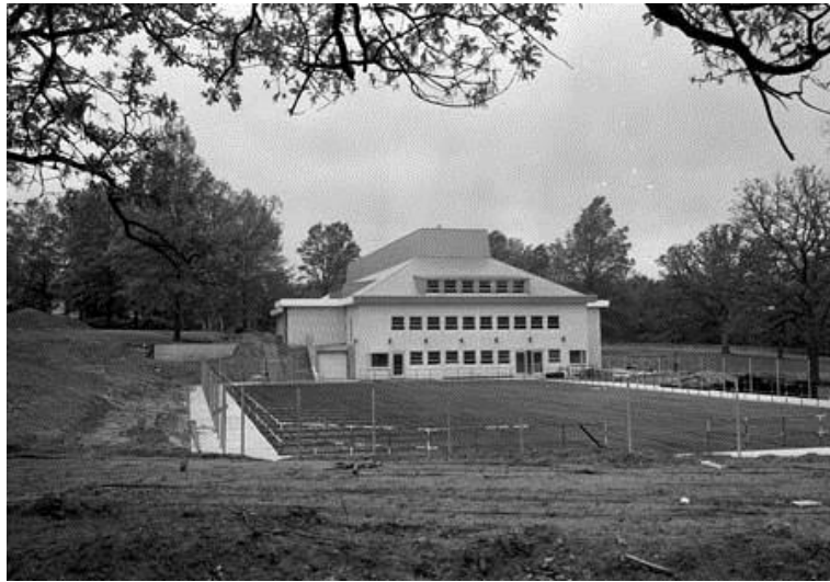
Ice Rink During Construction, 1966
